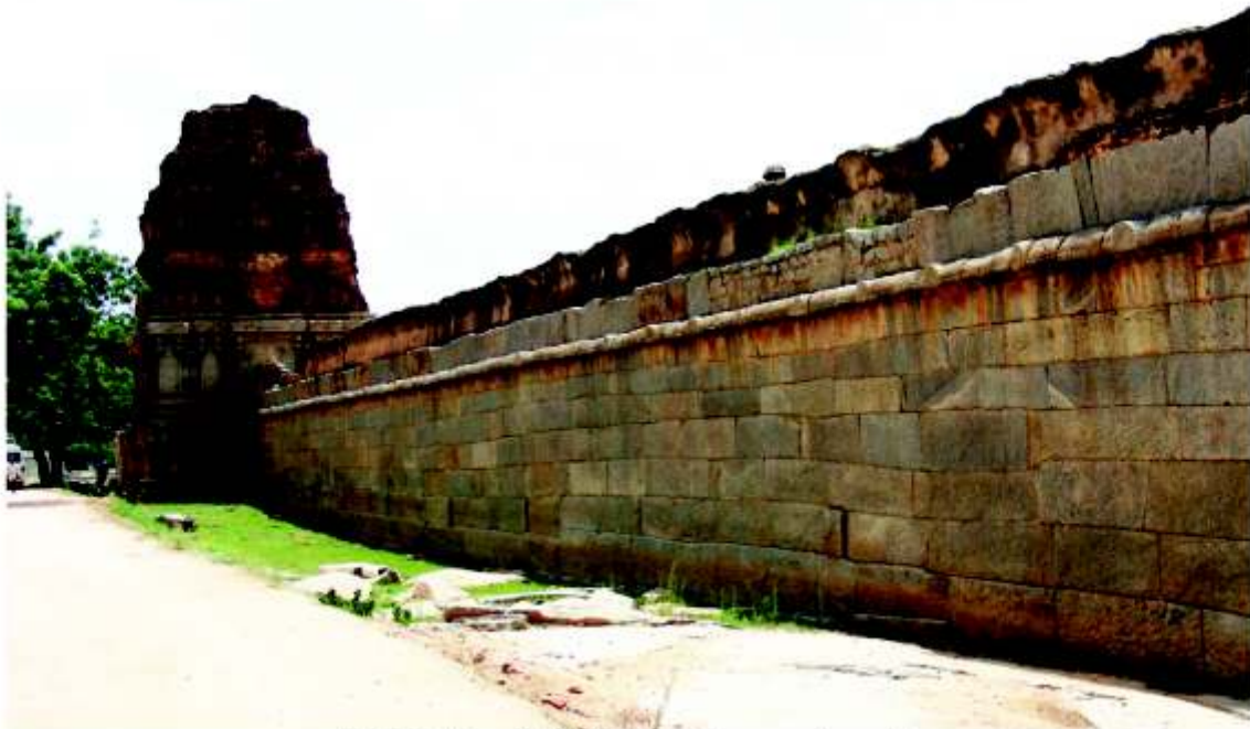
Fig.7 : Prākṛa wall with Southern Gopura , southern side
